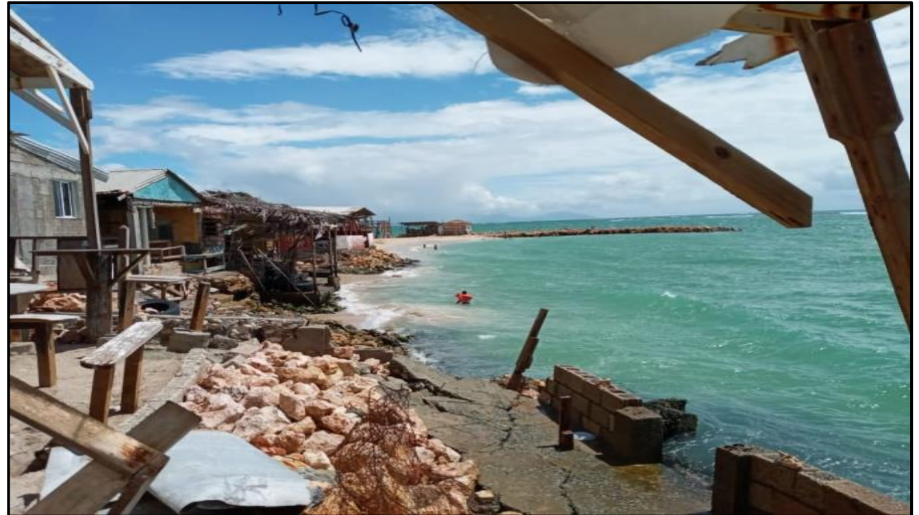
Remaining sections of a 'sea wall built by business owners. Source Andrew Bellamy 2020.
