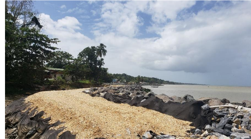
Cap de Ville Shoreline Stabilization Works (G2)
