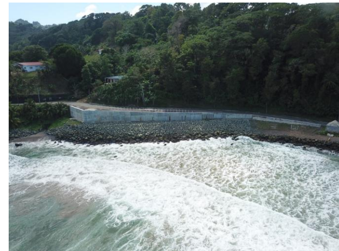
San Souci Shoreline Stabilization Works (C7)
