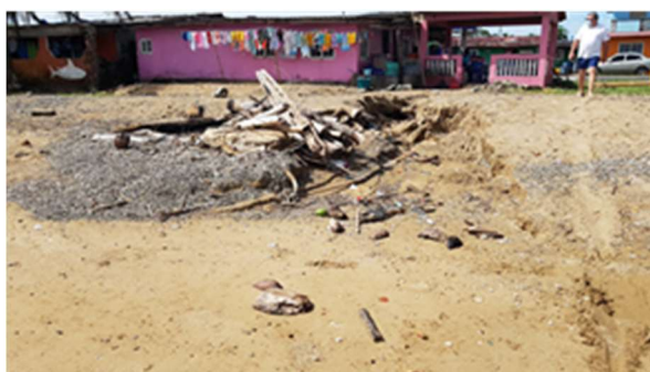
Photo 18. Erosion gullies due to poor storm drainage.
