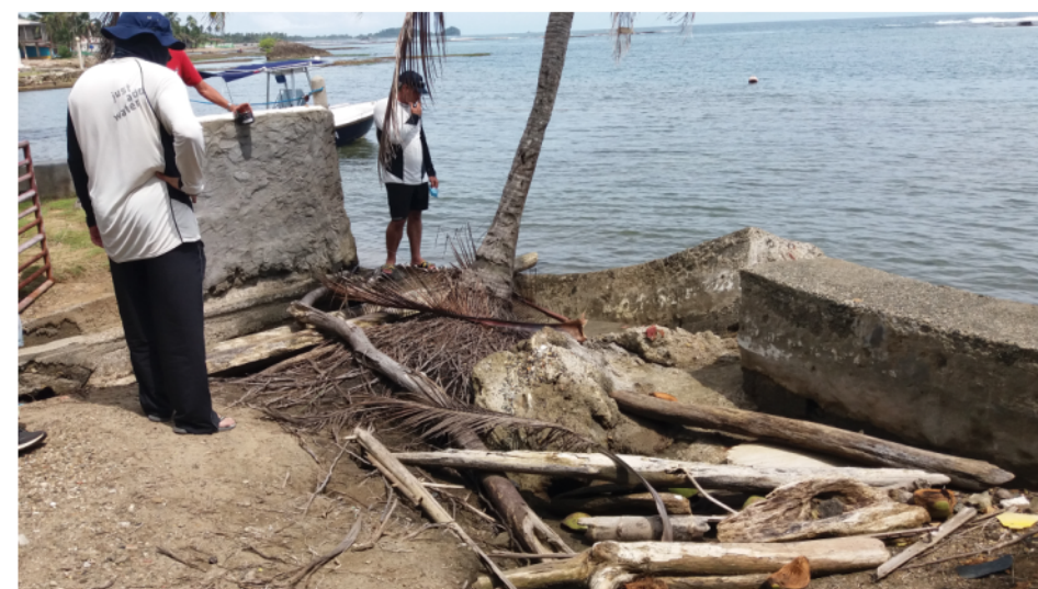
Damage by the action of the sea to the walls of protection to facilities
