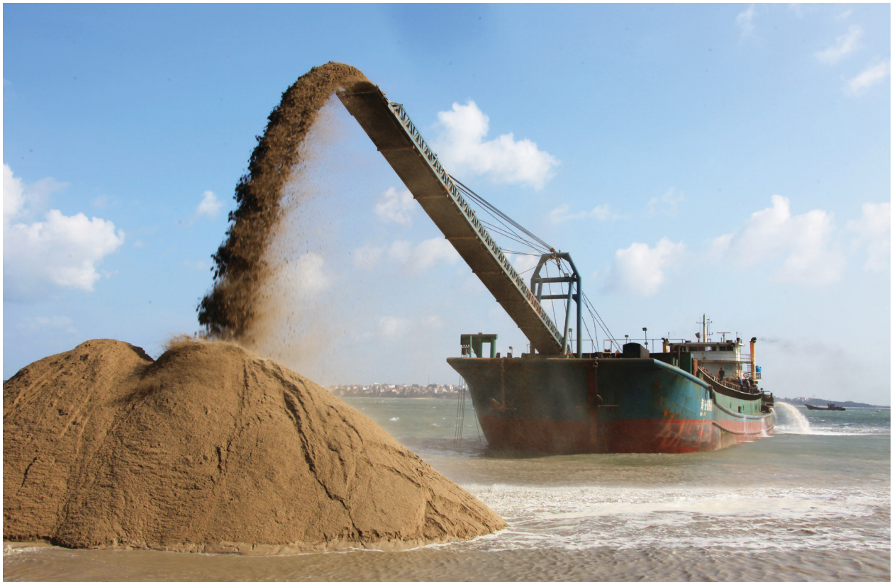
Figure 49 Feeding a beach with dredge
