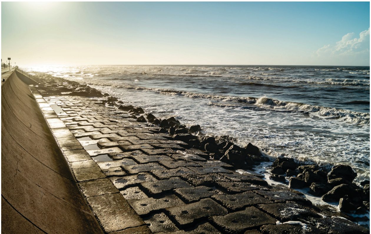
Figure 46. Curved face retaining dike
