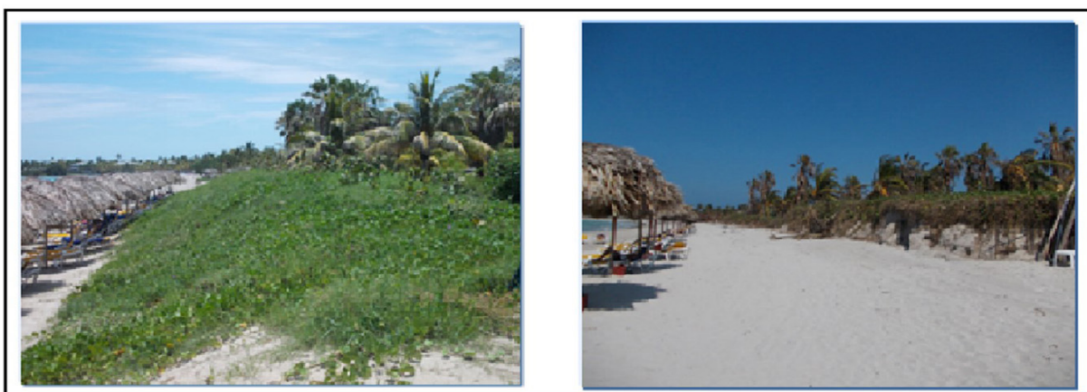
Figura 55 Left. Dune designed to protect the hotel from extreme erosive events and sea level rise. IberoStar Hotel. Varadero Beach, Cuba. July 2015. Right. A few days after Hurricane Irma in September 2017. (Juanes J. L.2017)
